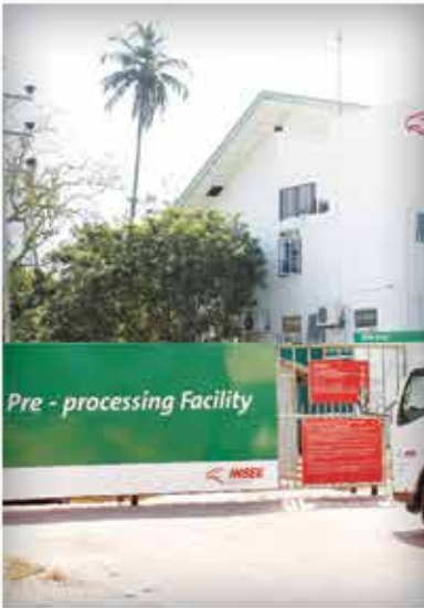
Ecocycle Pre-Processing Facility (PPF)
